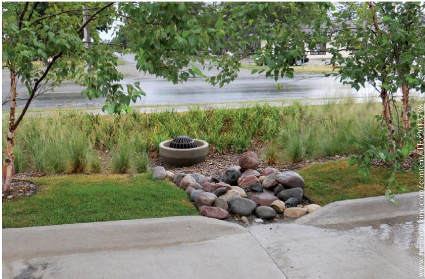
A pipe outlet structure with a grate (examples at the center of the photo above, and at the bottom of the photo at right) can be used to ensure a safe overflow for your vegetated swale.
