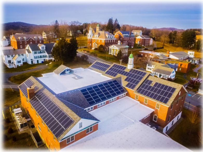
NST's 54 kW-DC solar array for Kimball Union Academy in Meriden, NH.
