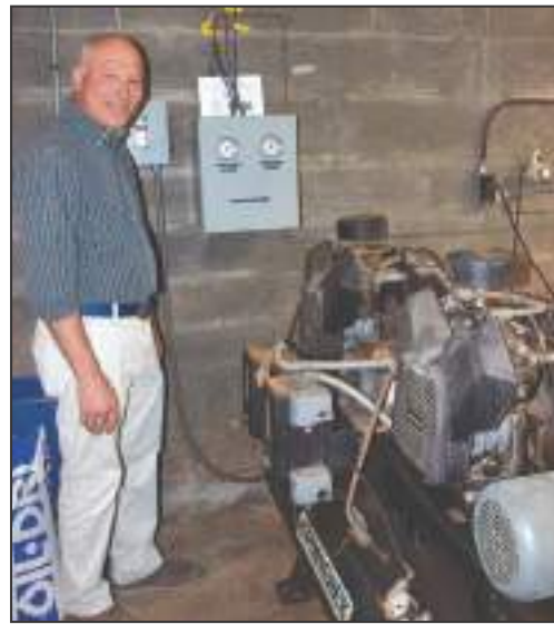
WCSU Building & Grounds Manager Joe Rigoli next to a pair of compressors that charge lines of pressurized air at WUHS/MS. He says the system is hugely wasteful because it is constantly running, unlike a more modern system that has fine controls. "It's basically the Stone Age," Rigoli said with a laugh, adding, "There is way more efficient technology out there."
