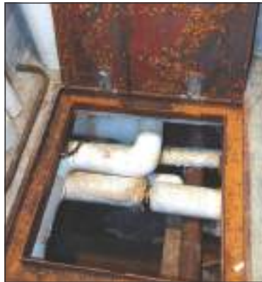
A hatch used to gain access to the pipes and steam tunnels at WUHS/MS. The hatch is only about 18 inches square, so in order to get replacement pipes through it, the pipes would either need to be cut into tiny pieces or larger holes would need to be drilled through the floor. The hatch door also shows signs of rusting due to leaking steam, which has occurred at various points throughout the building. Robert Shumskis Photo
