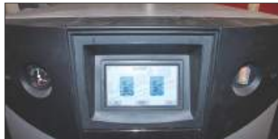
The control display on one of the LAARS Heating Systems boilers at the Prosper Valley School in Pomfret. There are two units and each is about the size of a refrigerator, as opposed to the unit at WUHS, which is several times larger. Robert Shumskis Photo
